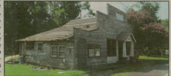
Crisfield-Somerset County Times/Richard Crumbacker The former store as it looked in late August 2018, just days before it was razed to make way for new construction.
