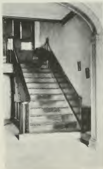
HALL AND STAIRWAY
