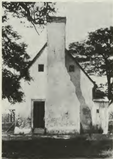
End View Showing Odd Chimney
