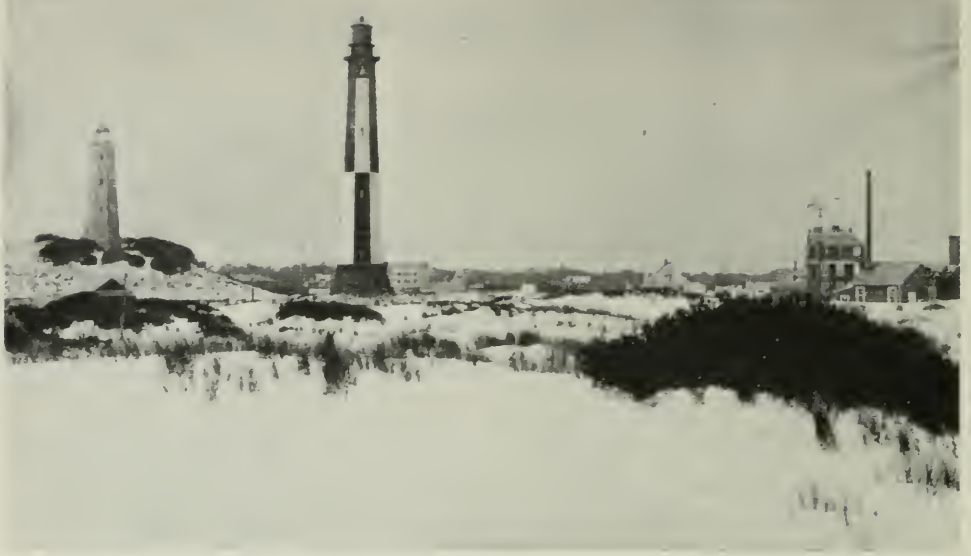
CAPE HENRY LIGHTHOUSE, BUILT 1881 Old Tower to Left Built 1791. Light of New Tower 157 Feet Above the Ocean and Visible 19 Miles
