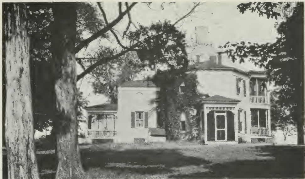
"CASTLE HAVEN" East End Showing Odd Brick Construction
