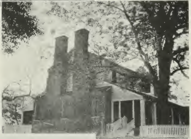
"DEEP FALLS" Thomas Homestead Note the Unusual Construction of Chimneys
